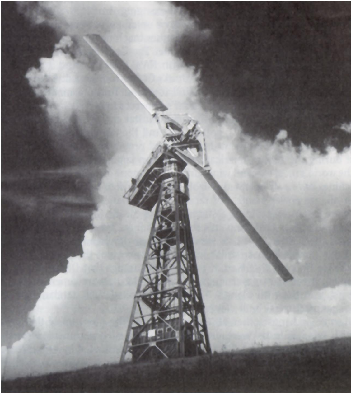
Figure 2.1: The 1.250 MW Smith-Putnam wind turbine. Reproduced from [35].
