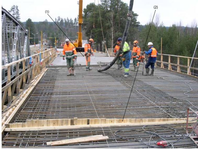
Figure 3.2: Casting of bridge Y288. (1) is the starting-point for the casting of the central part and (2) is the end-point. The starting-point and end-point are located 14.25 m from the ends of the bridge.
