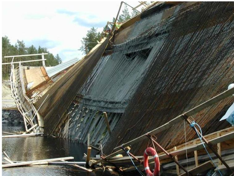
Figure 1.1: Bridge Y1504 over Gide älv after collapse (Courtesy of NCC AB).
